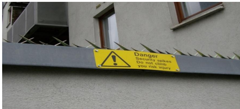
Figure 1: Spikes atop a barrier wall act as a deterrent to people trying to climb over the wall 3
